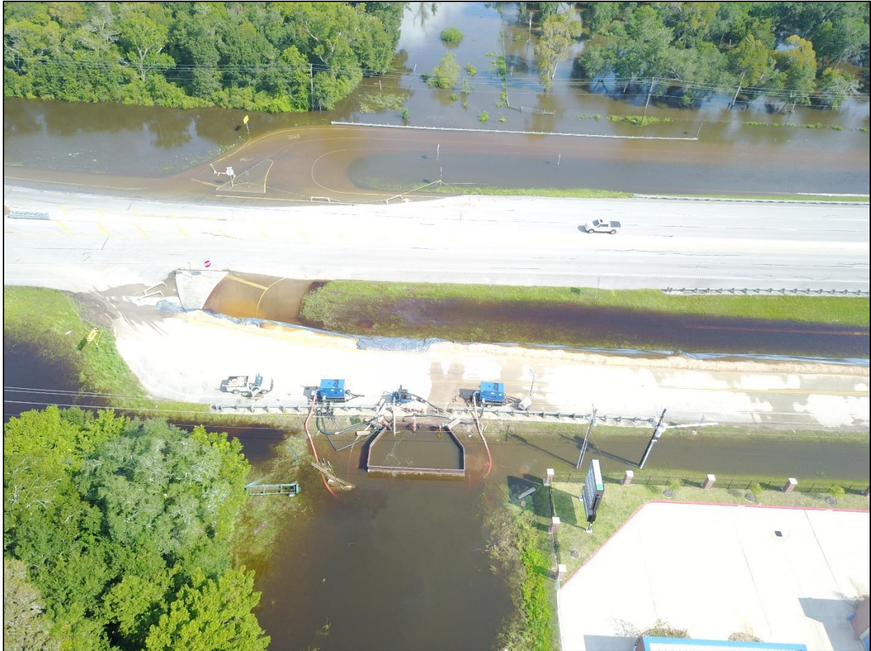
Figure 5e. Typically, water in the Brazos Canal (Slave Ditch) flows northward (from top to bottom in photo) from the south side of FM2004, through a set of three flap gates into a pumping chamber, through culverts under FM2004, and then northward to Bastrop Bayou (see Fig. 3). Note the three large blue pumps that are pumping water from the Brazos Canal and into the pumping chamber in order to force the water to flow northward through the culverts. The purpose of the flap gates is to prevent water from flowing from the north through the Brazos Canal and into the city of Lake Jackson when Bastrop Bayou is at flood stage. From noon on August 28, 2017, until 4:50 pm on August 31, 2017, one of the flap gates was stuck open at a 45° angle, which allowed water to flow southward out of the pumping chamber into the Brazos Canal south of FM2004. Based on the minimum drop in water level of one foot from the north to the south side of the flap gates (equivalent to the drop in water level from the inside to the outside of the pumping chamber), Grounds (2019) showed that water was flowing out of the pumping chamber southward into the Brazos Canal faster than it was being pumped into the pumping chamber. On that basis, the high water level in the pumping chamber resulted not from the pumping, but from the southward flow through the culverts. Still shot of drone video taken on or before September 3, 2017, and provided by Matías J. Adrogué, PLLC.
