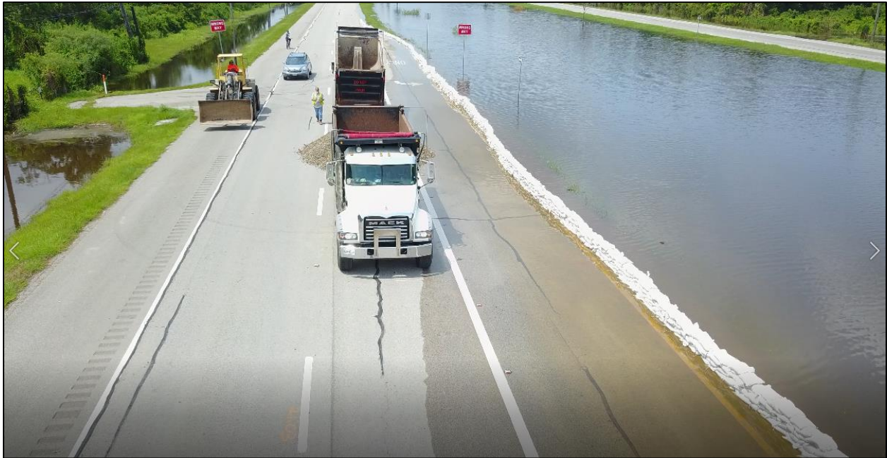
Figure 4b. A 24-inch high, 2000-foot long sandbag dam was constructed along the south side (eastbound lane) of FM2004 to prevent flooding of the city of Lake Jackson. View is looking west. Still shot at 1:00 of drone video labeled Before-8 taken on or before September 3, 2017, and provided by Matías J. Adrogué, PLLC.
