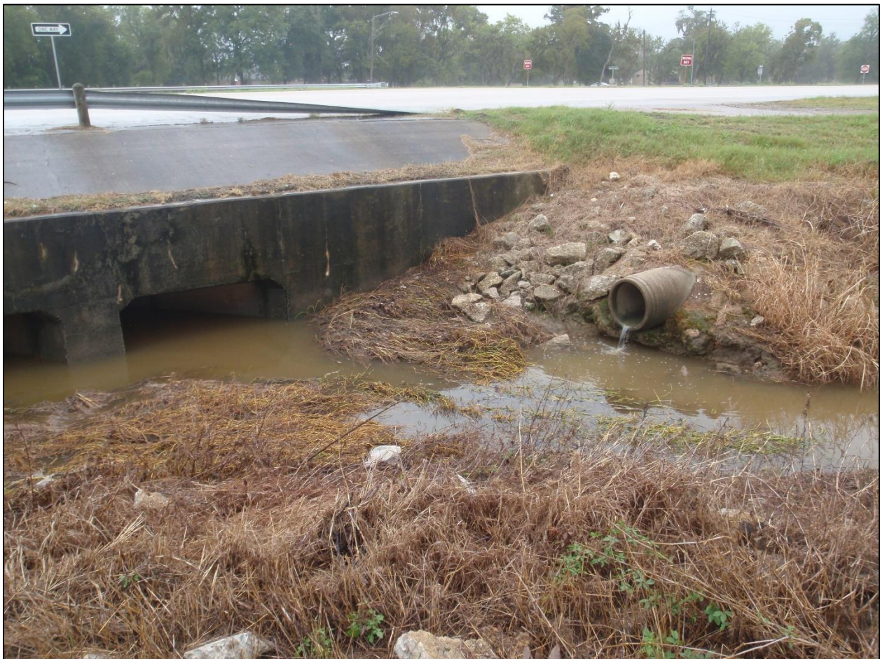
Figure 14b. Typically, water in the “East Ditch” flows from the south side of FM2004, through the culvert under FM2004, and then westward (toward the right in the photo) to Bastrop Bayou (see Fig. 3). However, after diversion by the sandbag dam, water most likely flowed eastward through the same ditch (see Figs. 10-11) and emerged on the south side of FM2004 (opposite side of highway in background of photo). View looking to the south. Photo taken by the author on October 30, 2019.
