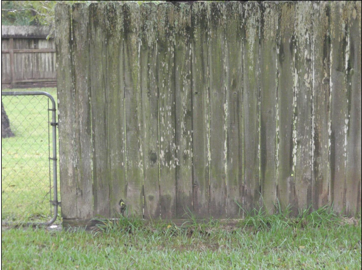
Figure 7b. The fence in the backyard of 12 Sherwood Drive (property of Kevin McKinney) just outside of Richwood shows a watermark below which light-grayish lichens were removed by the flood water. The average watermark along the fence was measured at 24 inches above the ground surface. Photo taken by the author on October 30, 2019.
