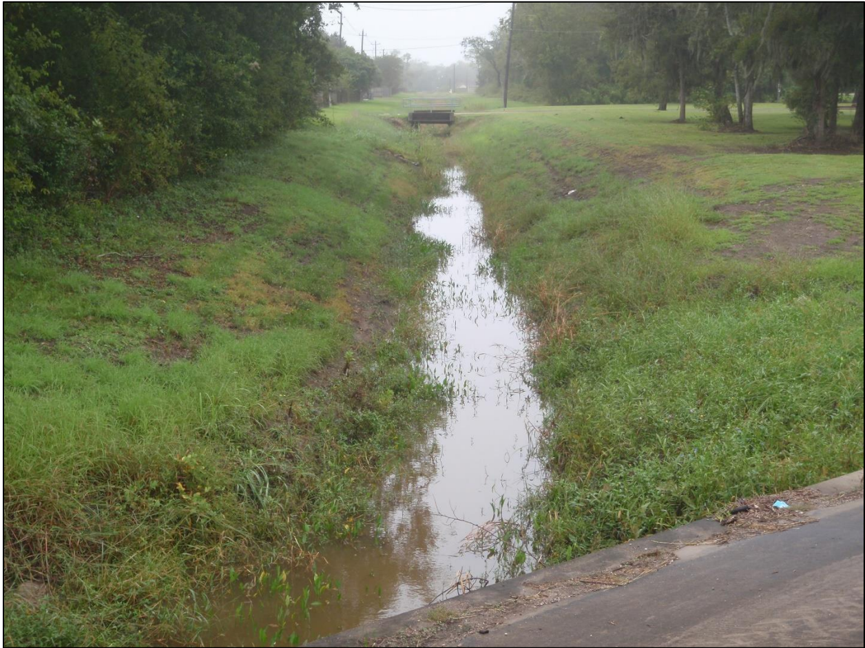
Figure 14c. Typically, water in the “East Ditch” flows northward (toward the viewer) from the south side of FM2004, through the culvert under FM2004, and then westward to Bastrop Bayou (see Fig. 3). View from the south side of FM2004 (note highway in foreground) looking to the south. However, after diversion by the sandbag dam, water most likely flowed eastward through the same ditch, through a culvert under FM2004, and emerged on the south side of FM2004 (see Figs. 10-11). The ditch is close to an interior boundary of the city of Richwood (Richwood on the right side of the photo). Photo taken by the author on October 30, 2019.
