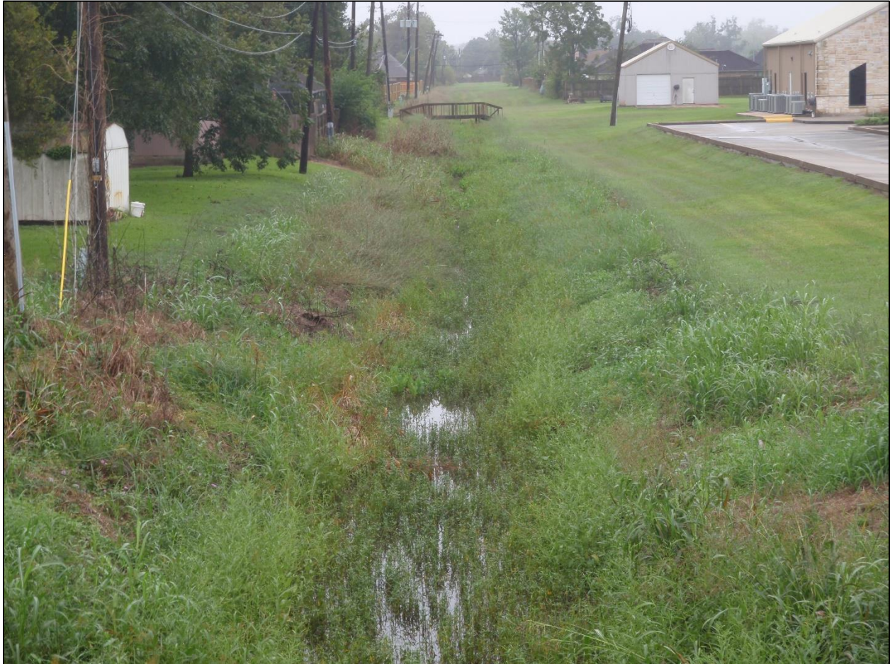
Figure 15b. Typically, water in the “West Ditch” flows northward (toward the viewer) from the south side of FM2004, through the culvert under FM2004, and then northward to Bastrop Bayou (see Fig. 3). View from the south side of FM2004 looking to the south. However, after diversion by the sandbag dam, water most likely flowed southward through the same ditch, through a culvert under FM2004, and emerged on the south side of FM2004 (see Figs. 10-11). The ditch is close to the boundary of the city of Richwood (Richwood on the left side of the photo). Photo taken by the author on October 30, 2019.
