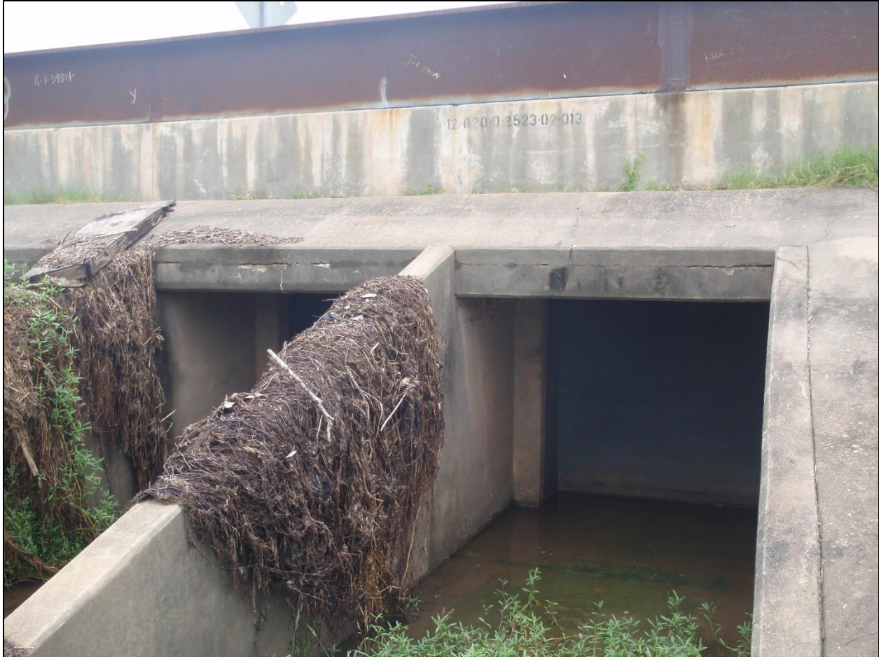
Figure 5b. Typically, water in the Brazos Canal (Slave Ditch) flows northward from the south side of FM2004 and through a set of three flap gates into a pumping chamber and then northward to Bastrop Bayou (see Fig. 3). View looking to the north. The purpose of the flap gates is to prevent water from flowing from the north through the Brazos Canal and into the city of Lake Jackson when Bastrop Bayou is at flood stage. From noon on August 28, 2017, until 4:50 pm on August 31, 2017, one of the flap gates was stuck open at a 45° angle, which allowed water to flow southward from Bastrop Bayou into the Brazos Canal south of FM2004. Photo taken by the author on October 30, 2019.
