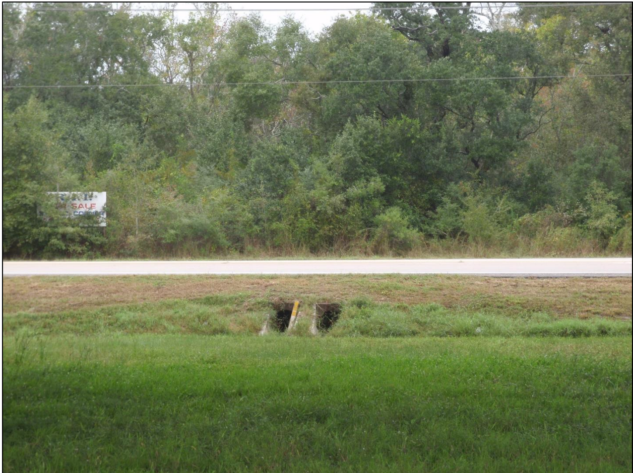
Figure 12. During the overflow from Bastrop Bayou, water most likely flowed southward through the culverts underneath the north side (westbound lanes) of FM2004 before ponding against the sandbag dam that was constructed on the south side (eastbound lanes) of FM2004 (see Figs. 3, 4a-c). View looking to the north under the FM2004 overpass over Old Angleton Road (see Fig. 3) from a site slightly west of the site of Fig. 4c. The median strip is visible in the foreground with the FM2004 north frontage road in the middle ground. Note that flood water mostly did not flow across FM2004, but flowed under the highway and ponded in the median strip (see Figs. 4a-b, 5e, 9). Photo taken by the author on October 30, 2019.
