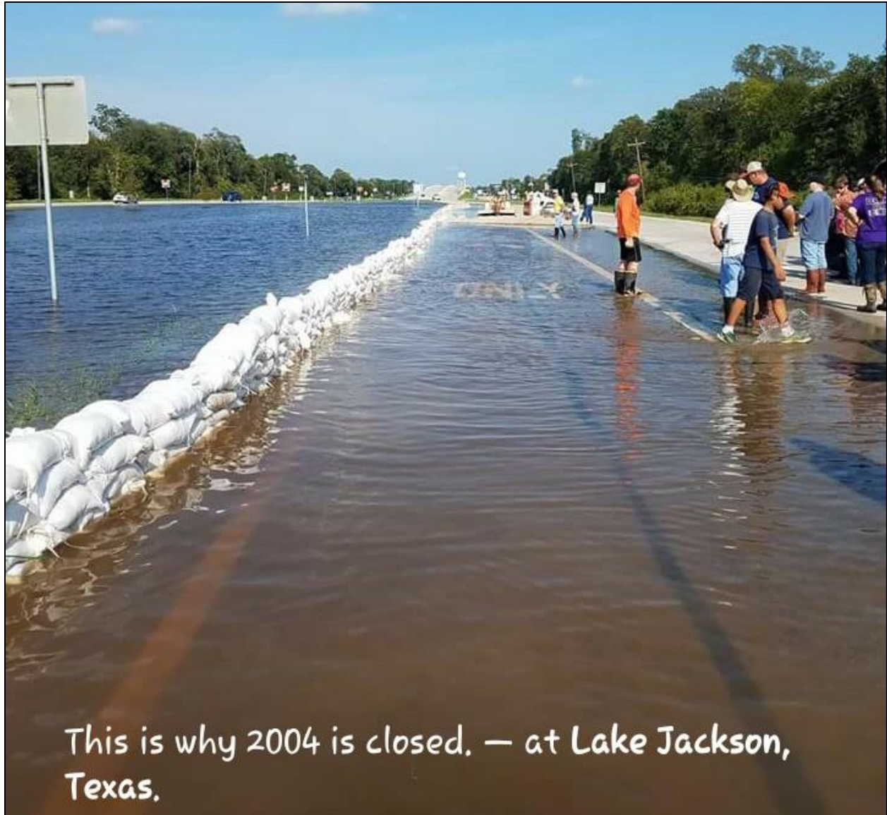
Figure 4a. A 24-inch high, 2000-foot long sandbag dam was constructed along the south side (eastbound lane) of FM2004 to prevent flooding of the city of Lake Jackson. View is looking east. Note FM2004 overpass over Old Angleton Road in background (see Fig. 3). Photo taken on or before September 3, 2017, and provided by Matías J. Adrogué, PLLC.
