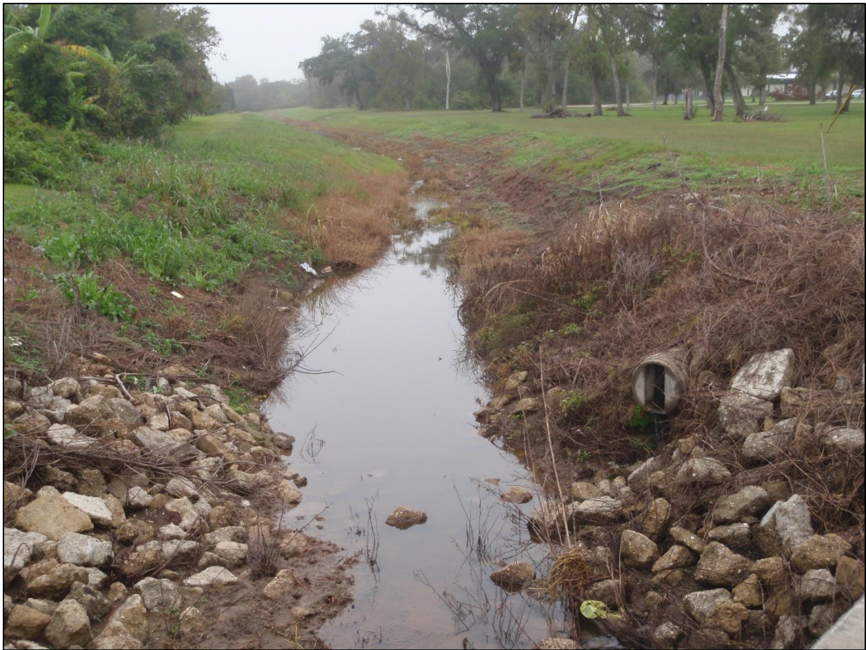
Figure 15a. Typically, water flows northward (away from the viewer) through the “West Ditch” to Bastrop Bayou (see Fig. 3). However, after diversion by the sandbag dam, water most likely flowed southward through the same ditch toward FM2004 (see Figs. 10-11). View from the north side of FM2004 looking to the north. Photo taken by the author on October 30, 2019.
