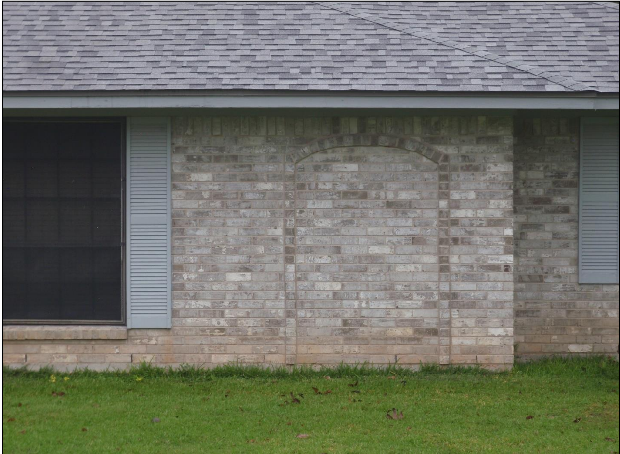
Figure 7a. Homes in Richwood and adjacent county areas that were not power washed after the flood still show watermarks about two feet above the ground surface. Photo shows the home at 14 Sherwood Drive. Photo taken by the author on October 30, 2019.
