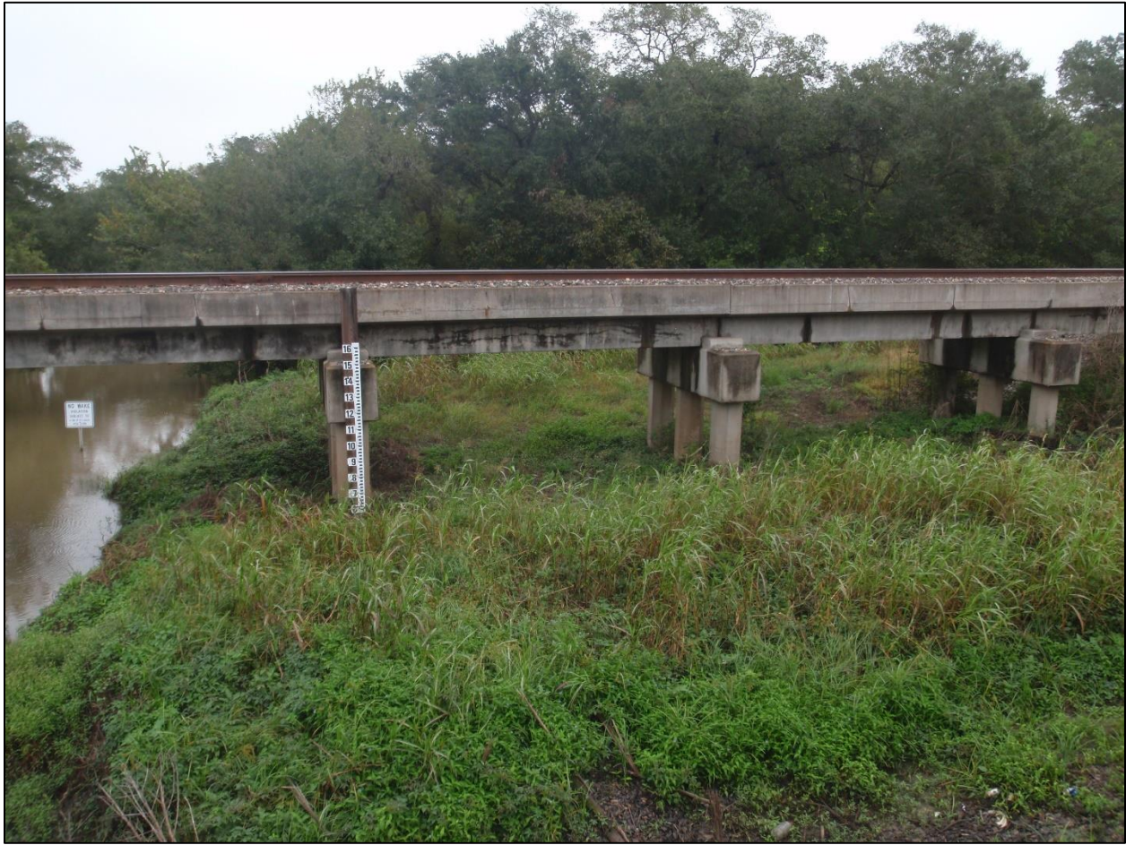
Figure 13. It is most likely that the flood water crossed the railroad under the bridge over Bastrop Bayou on the south side (right side of photo) of the bayou (see Figs. 10-11). View looking downstream to the east. Note the stream gage bolted to the bridge. Photo taken by the author on October 30, 2019.
