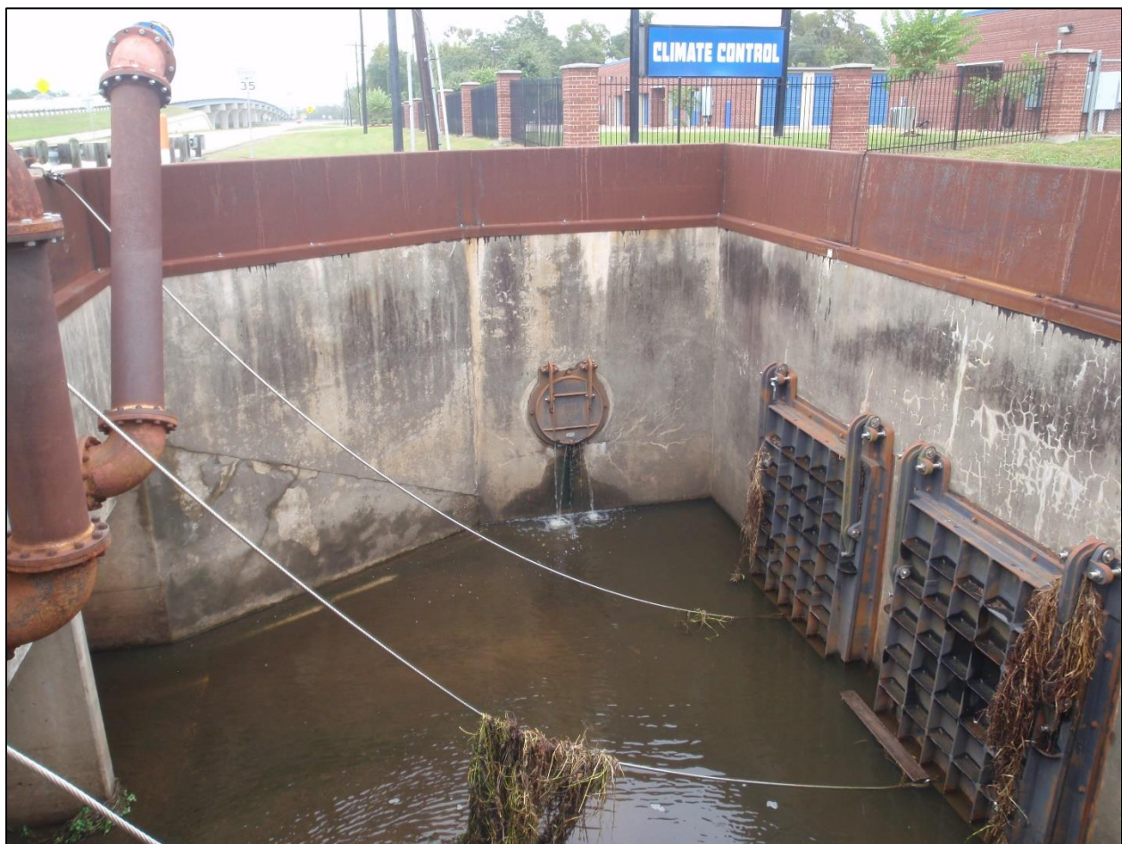
Figure 5c. Typically, water in the Brazos Canal (Slave Ditch) flows northward from the south side of FM2004, through a set of three flap gates into a pumping chamber, through culverts under FM2004, and then northward to Bastrop Bayou (see Fig. 3). View looking to the east. The purpose of the flap gates is to prevent water from flowing from the north through the Brazos Canal and into the city of Lake Jackson when Bastrop Bayou is at flood stage. From noon on August 28, 2017, until 4:50 pm on August 31, 2017, one of the flap gates was stuck open at a 45° angle, which allowed water to flow southward from Bastrop Bayou into the Brazos Canal south of FM2004. Note the cables for manual opening of the flap gates, the pipes on the left side for direct pumping into the Brazos Canal on the opposite (north) side of FM2004 (see Fig. 5d), and the FM2004 overpass in the left background (see Fig. 3). Photo taken by the author on October 30, 2019.
