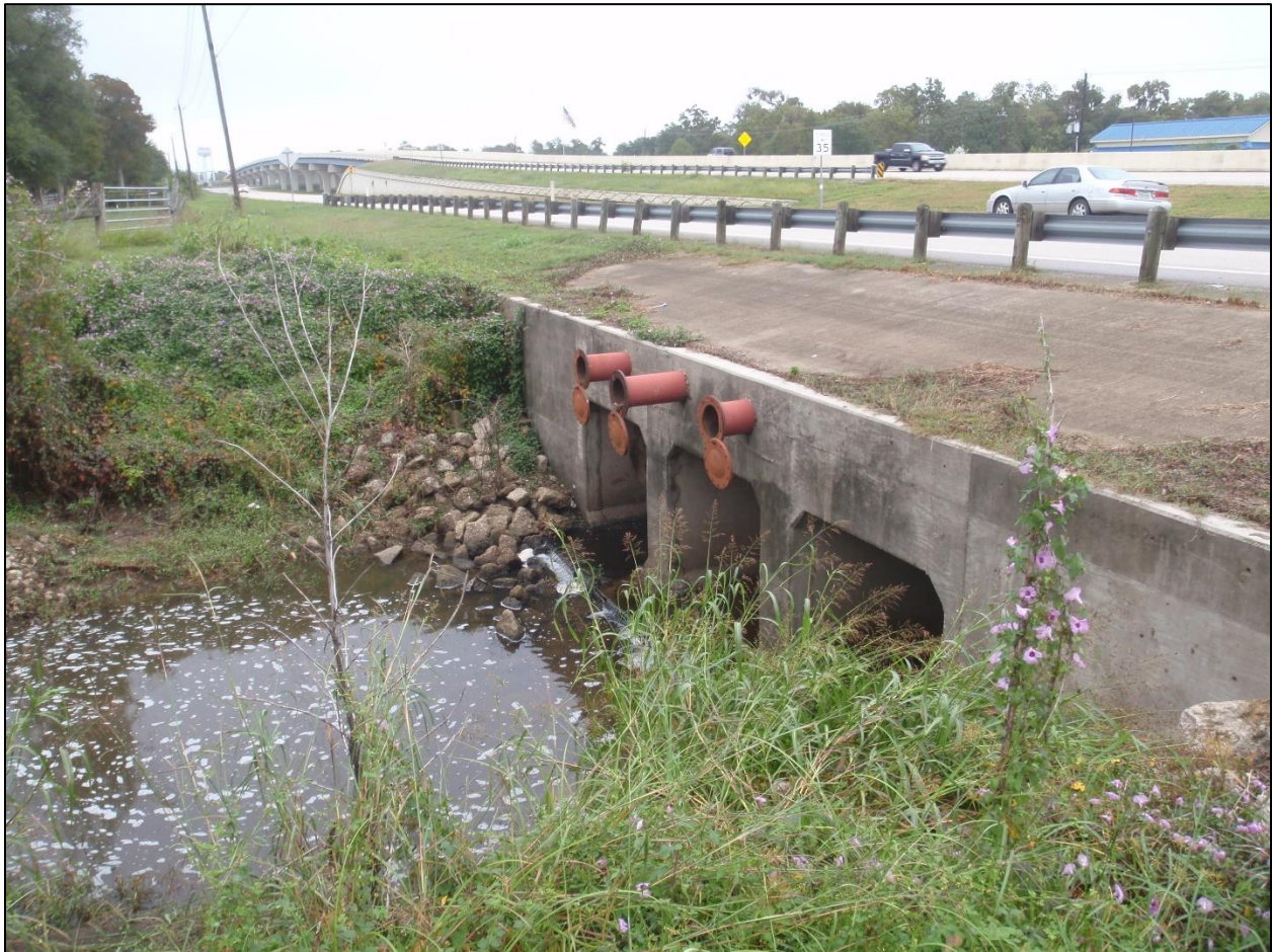
Figure 5d. Typically, water in the Brazos Canal (Slave Ditch) flows northward from the south side of FM2004, through a set of three flap gates into a pumping chamber, through culverts under FM2004, and then northward (to the left of the photo) to Bastrop Bayou (see Fig. 3). View looking to the east on the north side of FM2004. The purpose of the flap gates is to prevent water from flowing from the north through the Brazos Canal and into the city of Lake Jackson when Bastrop Bayou is at flood stage. From noon on August 28, 2017, until 4:50 pm on August 31, 2017, one of the flap gates was stuck open at a 45° angle, which allowed water to flow southward (to the right of the photo) from Bastrop Bayou into the Brazos Canal south of FM2004. In addition to the culverts, note the three pipes for direct pumping of water into the Brazos Canal (see Fig. 5c). Photo taken by the author on October 30, 2019.
