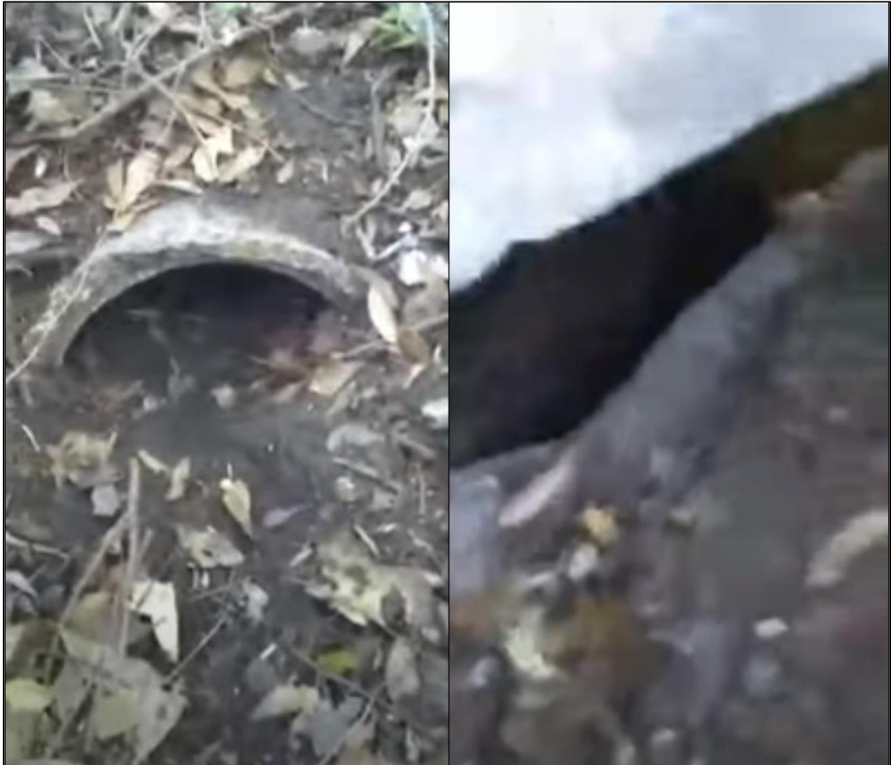
Figure 1. The left-hand photo shows a view to the southeast of an 18-inch stormwater pipe that is three-quarters blocked with mud and dead vegetation on the northwest corner of Flint Street and Central Park Road (see Fig. 2). The right-hand photo shows a view down the corresponding stormwater drain on Central Park Road that shows no water in the stormwater pipe. If the stormwater pipe were not blocked, presumably stormwater would flow to the southeast under Central Park Road (see Fig. 2). The left-hand and right-hand photos are stills from 0:16 and 0:34 of the video “Zeke just found another blocked pipe under Central Park Road” taken on April 22, 2021 and available online at https://www.youtube.com/watch?v=htGCOtyAThA .
